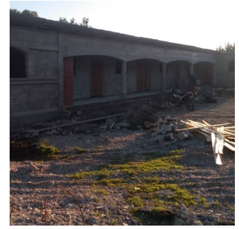
In progress construction
