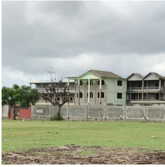
IMR prior to the earthquake
