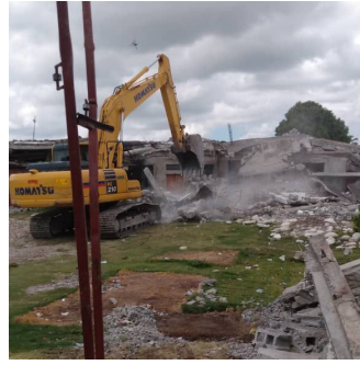
Clearing the rubble
